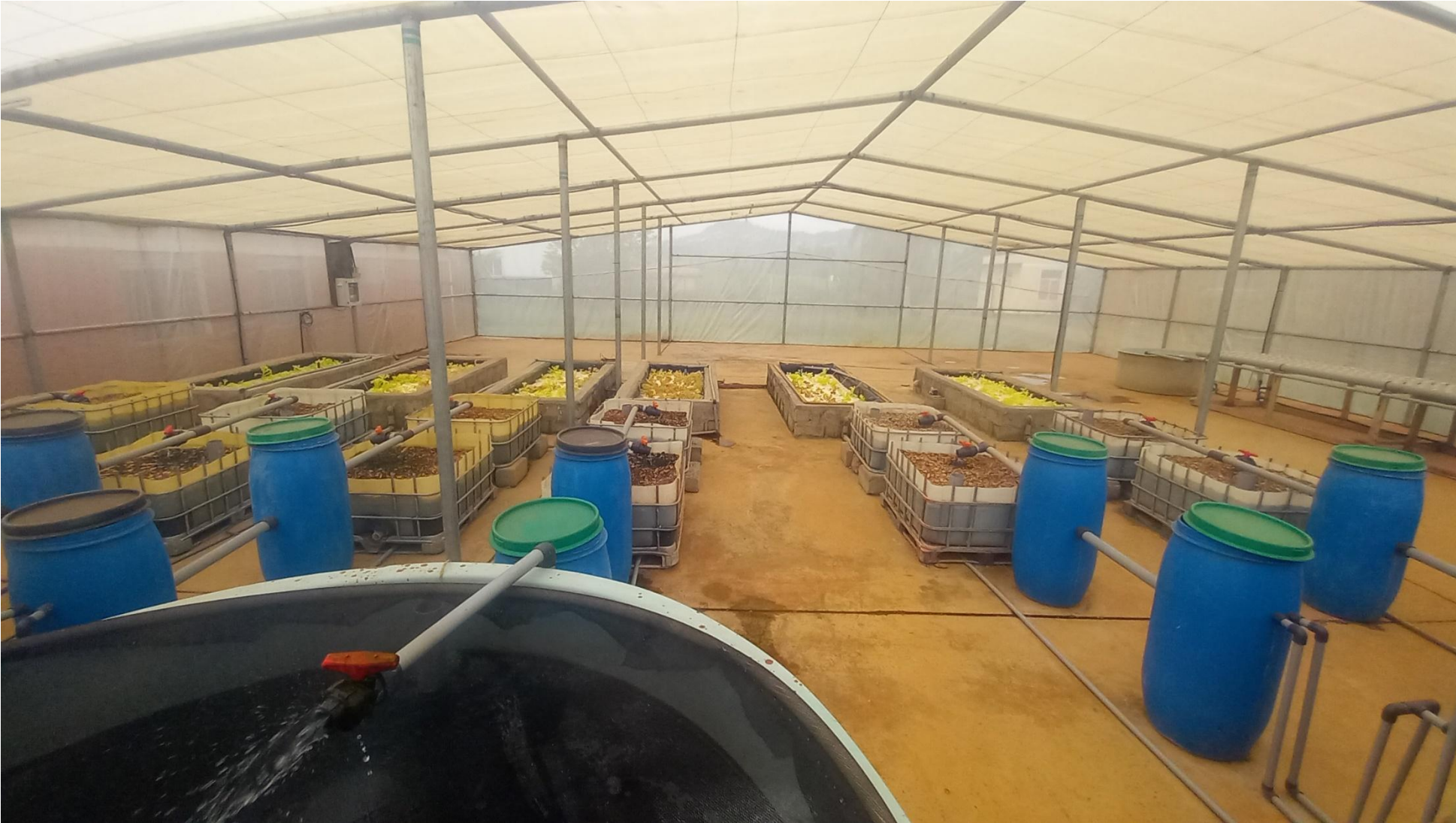
Figure: completed installation of the aquaponics system
