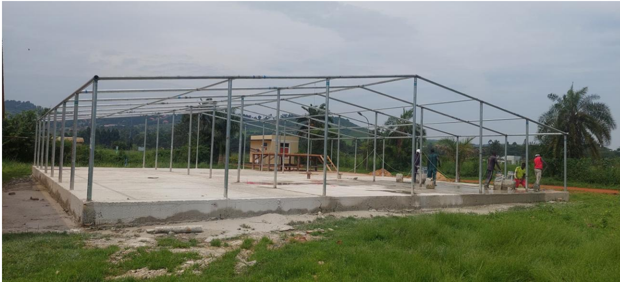
Fabrication, fixing of structural horizontal steel frames and the top, installation of internal structures
