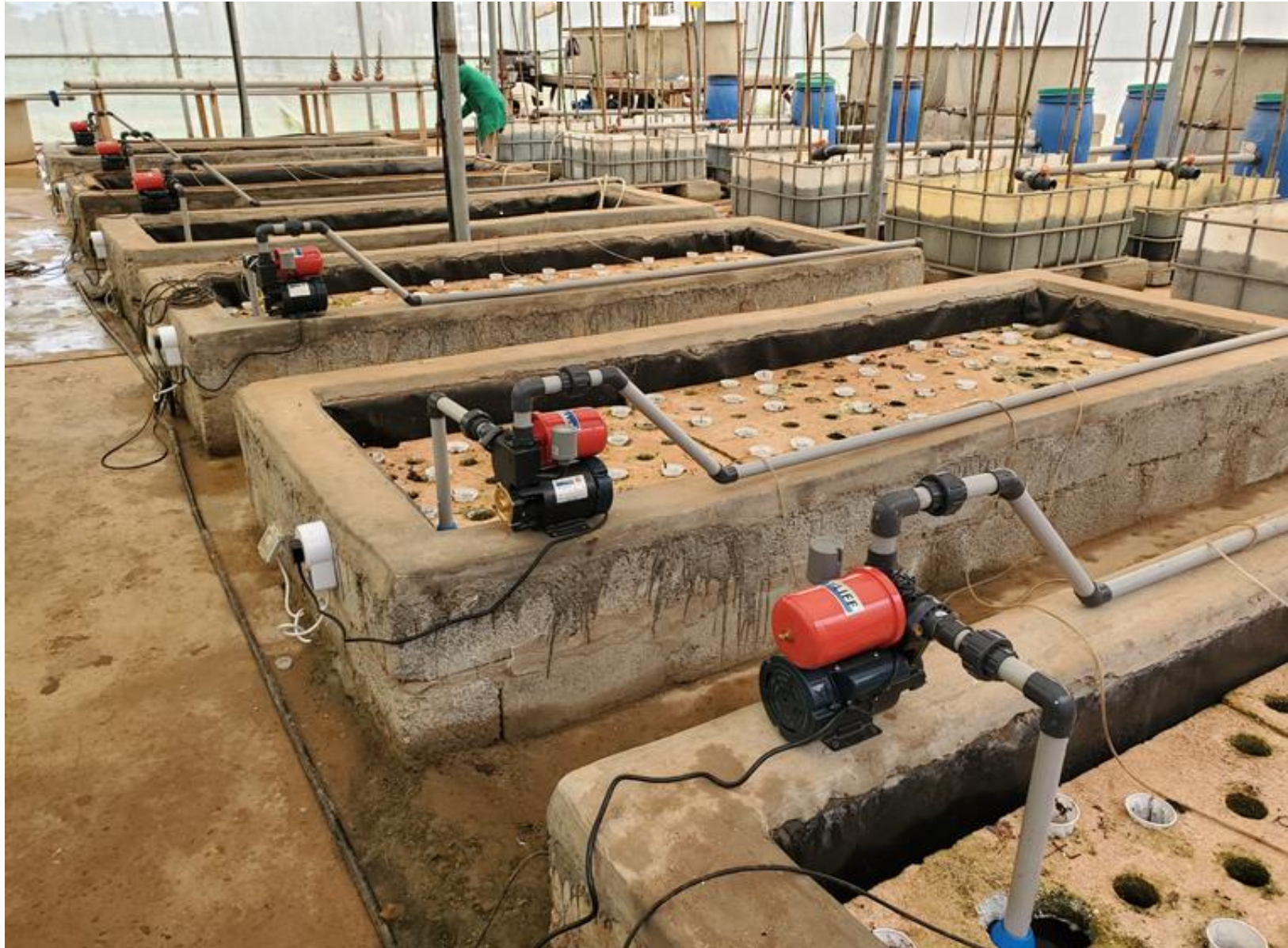
Figure: Repair and replacement of the water pumps is part of the maintenance
